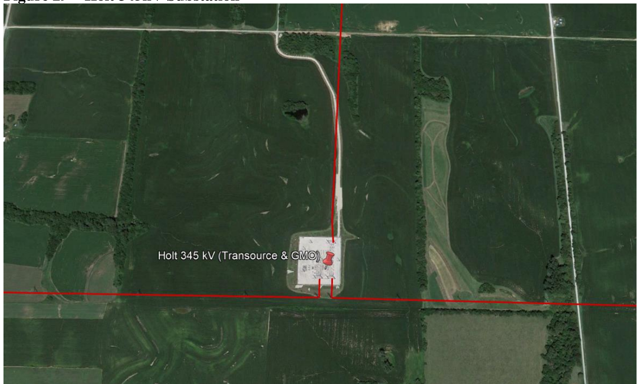
Figure 29 – Holt 345kV Substation
